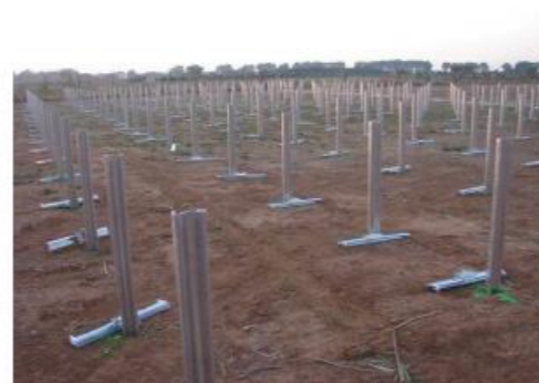
Aspect des supports
